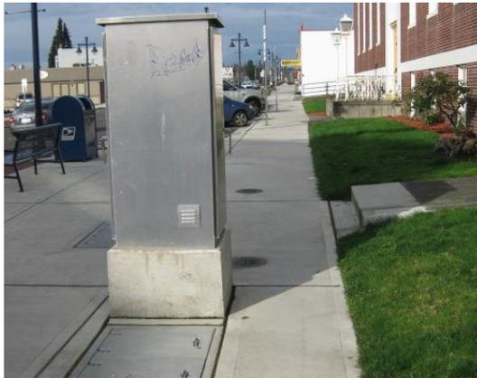
The electrical services for lights and other uses require a cabinet to house the electrical meter. The housing serving the post office area of the project was installed at the edge of the sidewalk near 6<sup>th</sup> Street. Visually, it appears out of place. The sidewalk in the area meets ADA requirements. Access to the panel is required from the back so it could not be located at the edge of the right of way. Other panels installed for this project are in less obstructive locations.
