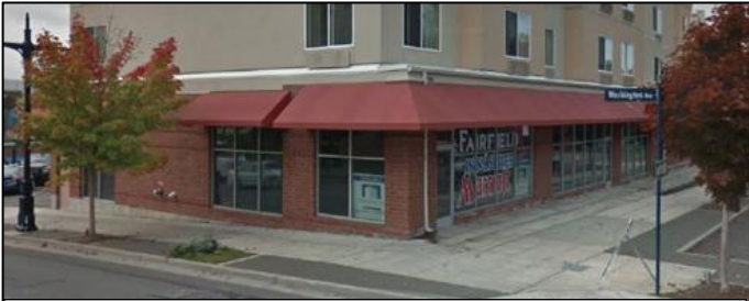
Existing façade on 4 th St and Washington Ave. Empty since construction in 2009
